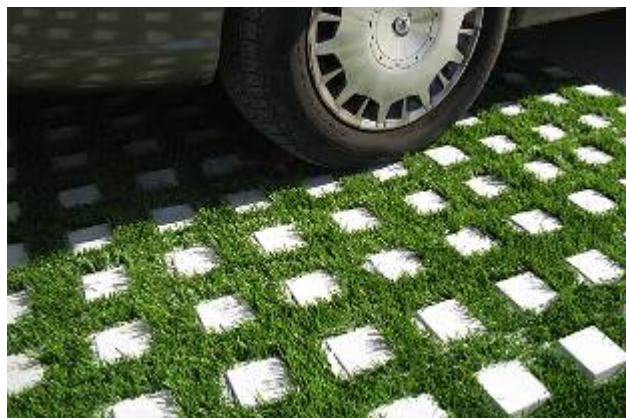
Figure 20: Integrating paving and soft landscape: (left) natural stone in lawn, (right) reinforced grass using 'Checker Block' concrete modular product.
