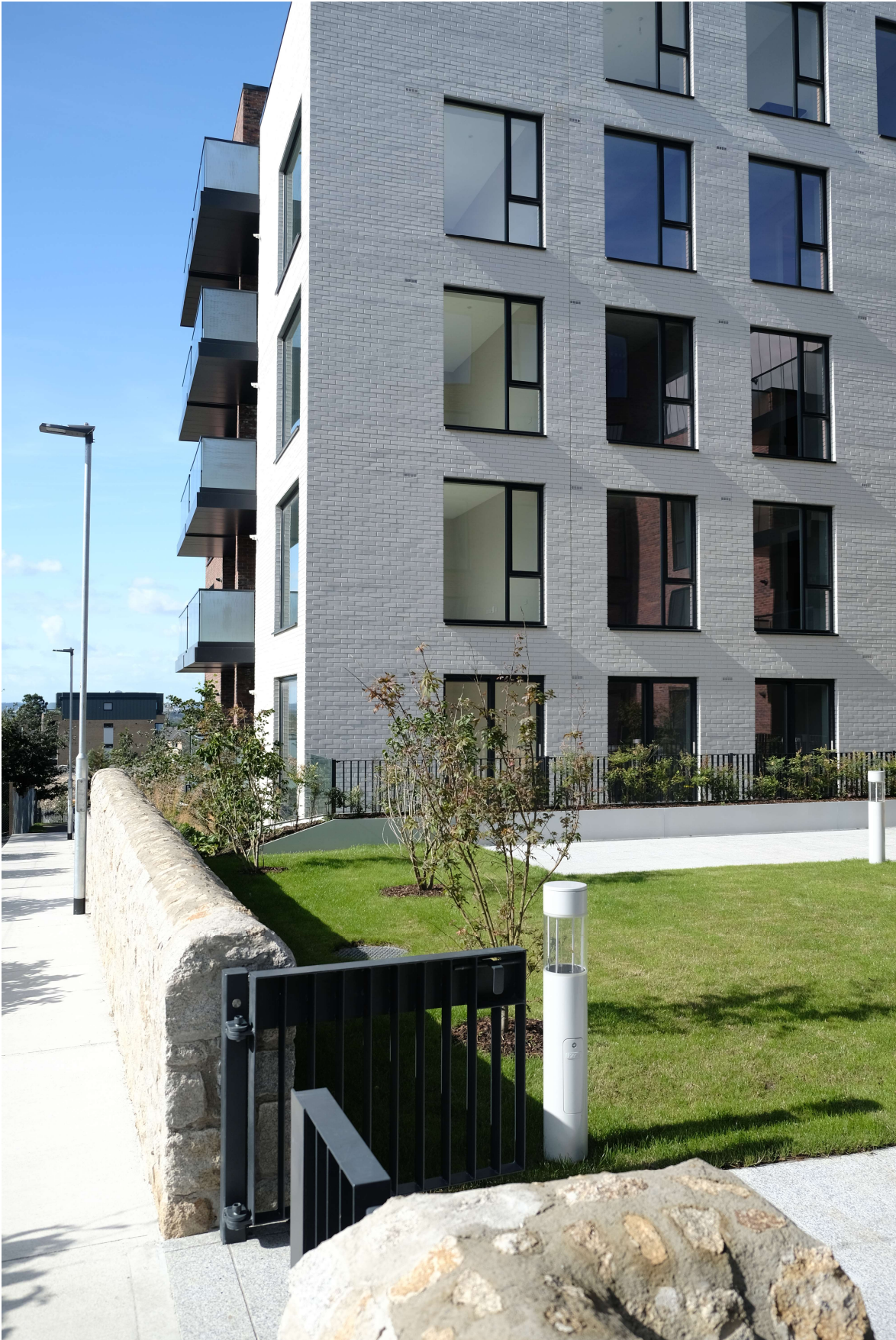
Figure 5: View from the site to the south looking along the edge of completed Phase 1 works.
